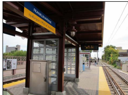
Hiawatha LRT Station at Franklin Avenue
