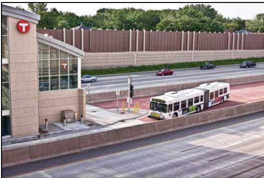
I-35W BRT Station at 46th Street
